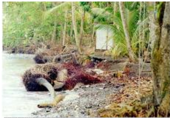
Erosion along the St. Margaret's Bay Coast
