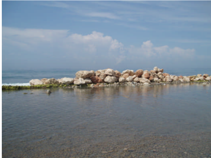
Limestone boulders placed on beach rock (at far left) at the Palisadoes narrow spot
