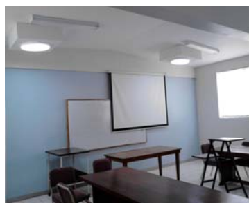
Seminar room with Solatube lighting fixtures
