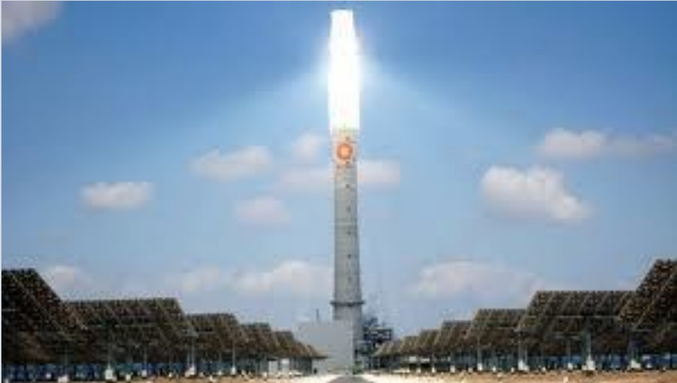
Sun's energy concentrated by mirrors Concentrated solar Power (CSP)
