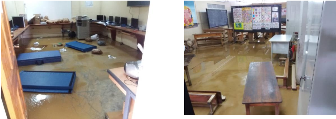
Figure 3 Damaged premises of St. Helena Hindu Primary School in 2018 October Flood
