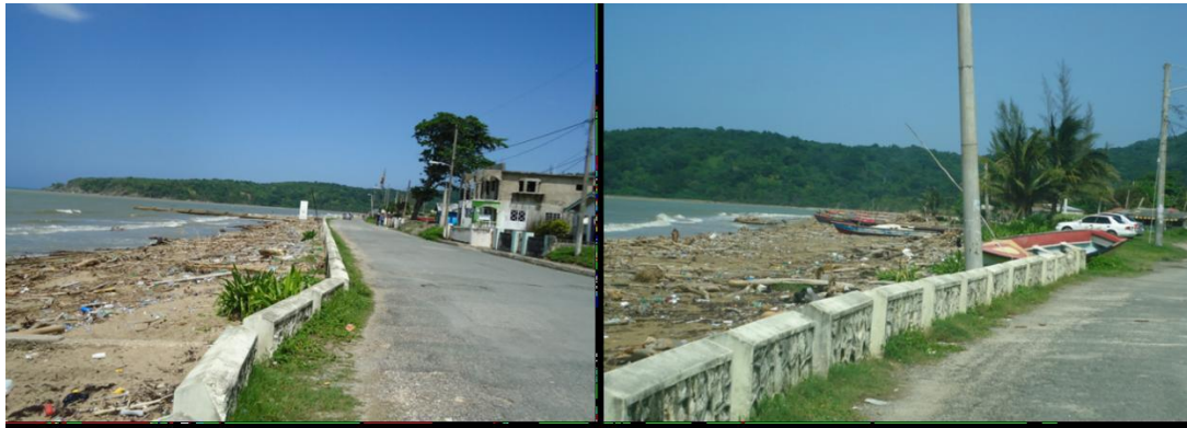
Figure 6 Debris deposits due to flooding – Port Maria Beach, May 2017
