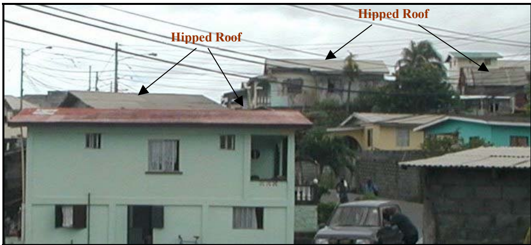
Photo 4.1 Housing and roof structure in the study areas in St Vincent
