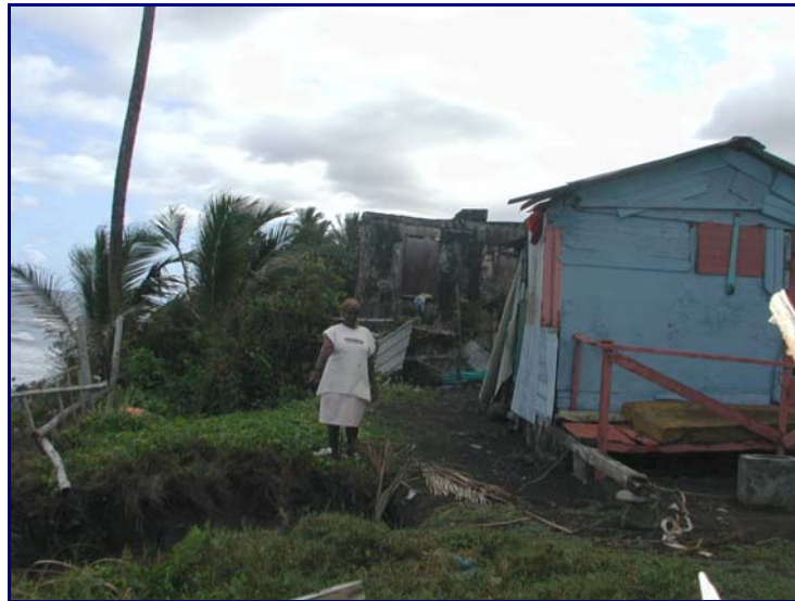
Photo 5.1. Erosion in Georgetown along the coast after hurricanes. Ferdinand 2005
