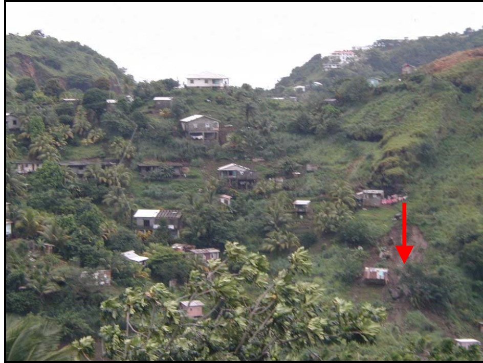
Photo 2.1: Squatter settlement on hillside in St Vincent, note the slippage which occurred after heavy rain during the 2005 hurricane season.
