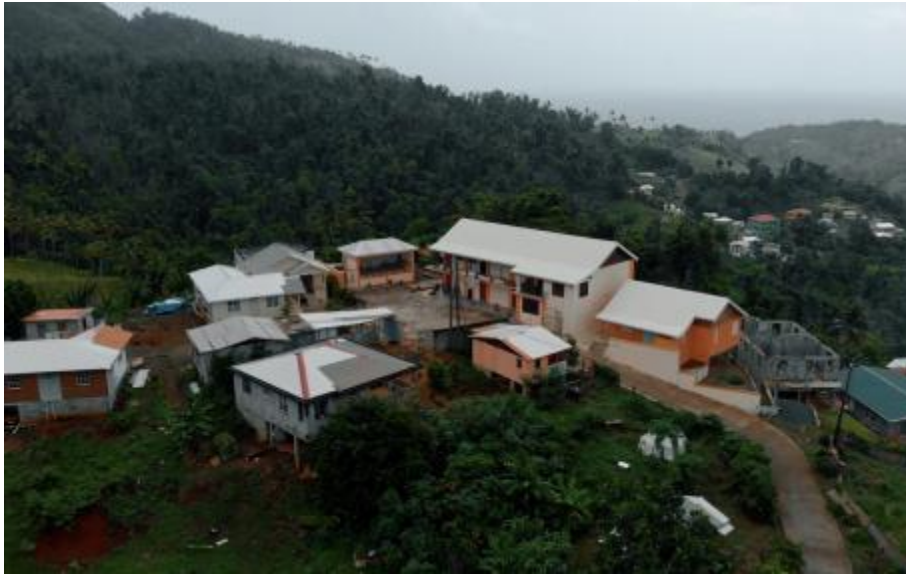
A school in Dominica rebuilt after Hurricane Maria. Photo by Tom Kucy/Clara Lionel Foundation.
