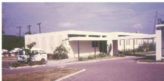
Fig. 4: The original Sickle Cell Clinic Building which opened in 1988.
