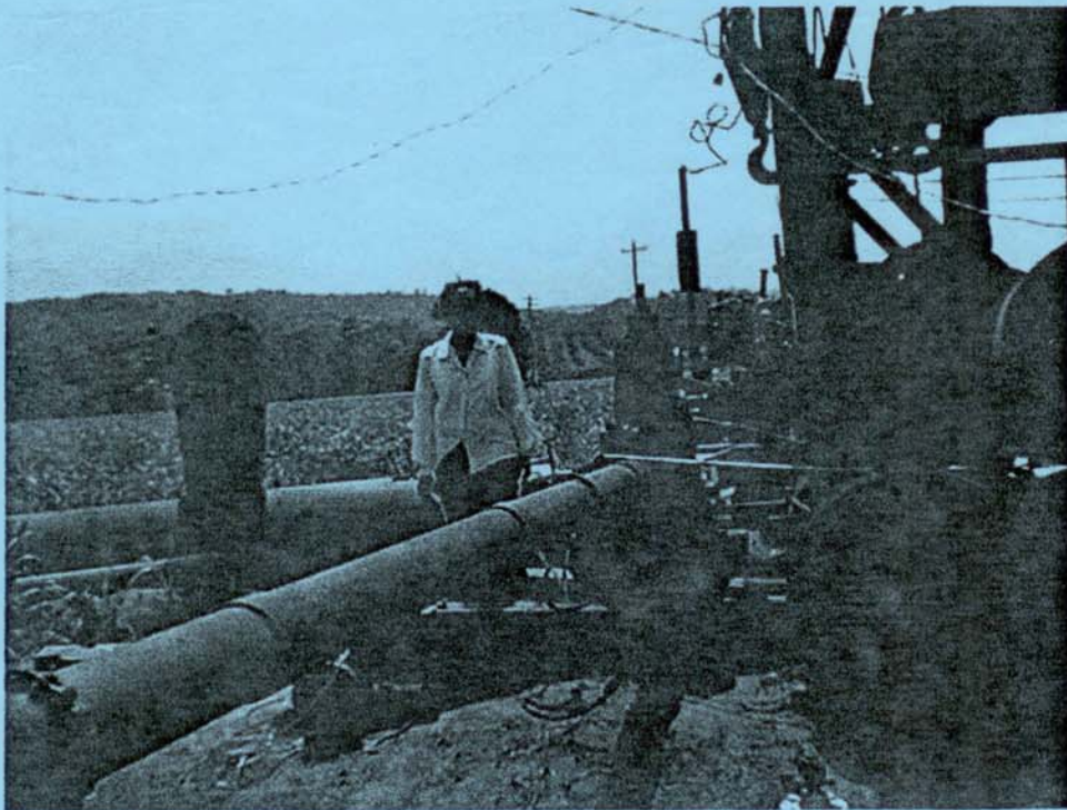
Well drilling at Low Ground, Clarendon
