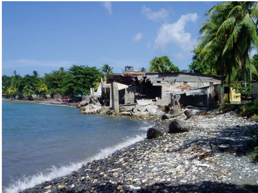
The results of severe erosion of the Jamaican coastline
