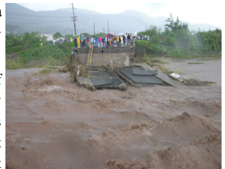
Residents remained isolated as the Harbour View bridge collapsed under the pressure of the Hope river. The bridge leads to the eastern side of the island
