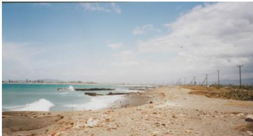
Figure 14. The Palisadoes groynes as they appeared before Hurricane Ivan, in July, 2002 (photo, Marine Geology Unit).
