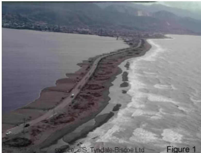
Figure 1. Aerial view of the narrow part of Palisadoes, looking towards Harbour View, taken just after Hurricane Ivan (photo, J.S. Tyndale-Biscoe Ltd.)
